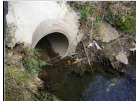
Stormwater pipe entering Neshannock Creek in New Castle
