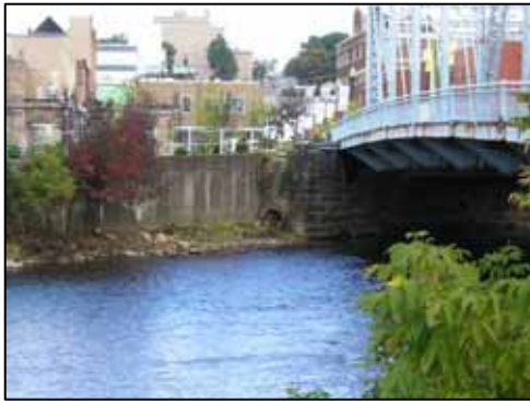
Neshannock Creek in New Castle: stormwater discharge, channelized stream, high percentage of impervious cover
