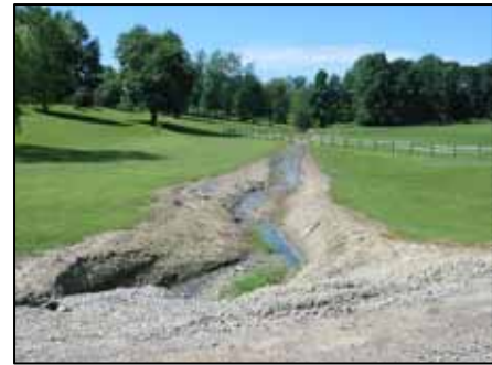
Erosion along a streambank in Lawrence County
