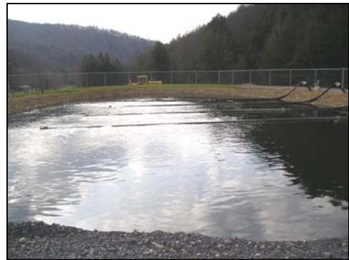
Example of a community sewage treatment system in Broad Top Township, Bedford County, PA
